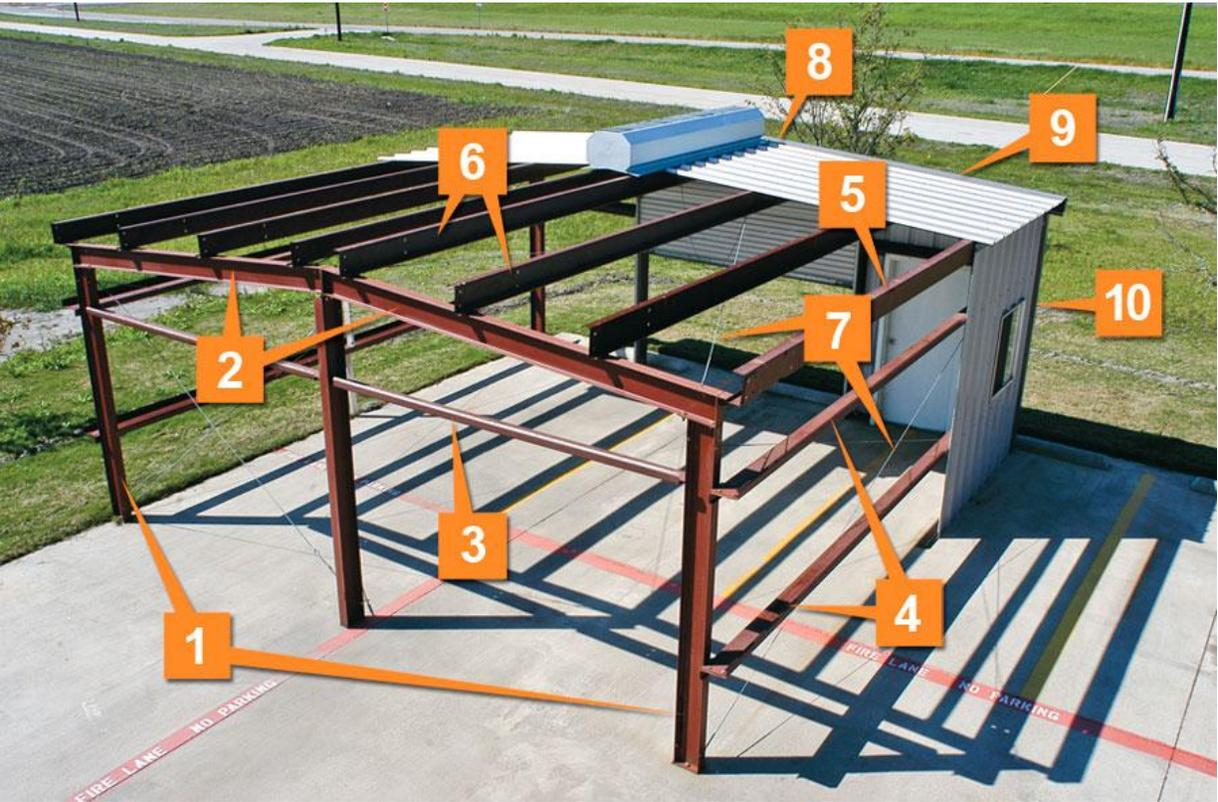
1. **Endwall Columns:** These are found at either end of the building and are the primary support structures for the endwalls, and in some case the entire building. Depending on the width of the building, there may be several columns.
