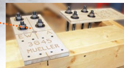
Anchor Bolt Templates
